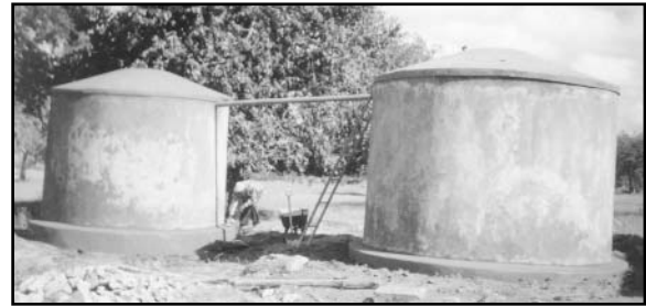
Catchment tanks to capture rainwater.
